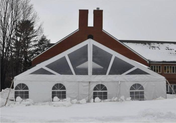
**BATTENING** is the process of securing the bottom of tent sidewall in an effort to minimize drafts. It is necessary to maintain temperature inside the tent. Sidewall designs using slide-track (keder) connections are also an option that will minimize drafts and wind.
